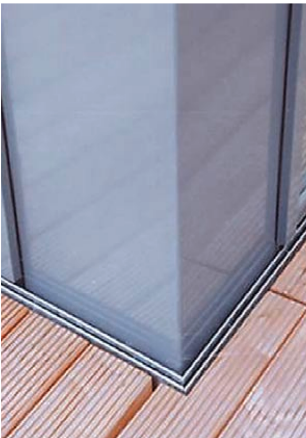
Asymmetrical slotted channels for draining a façade.
