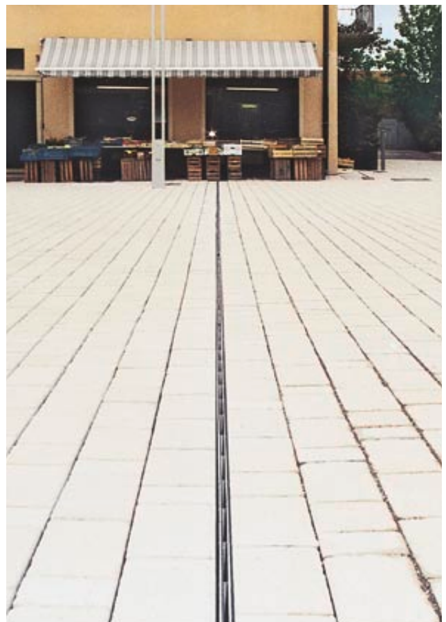
Symmetrical slotted channels for surface draining integrate unobtrusively into the slab paving.
